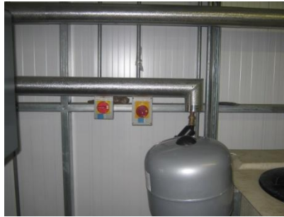
RWHS Cold water pump
