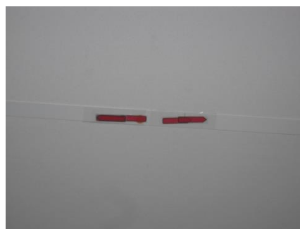
Marking on ceiling where valves are (above piano)
