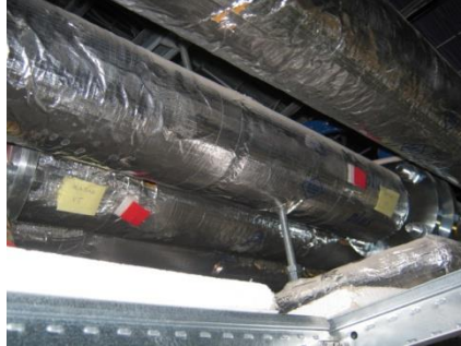
Hot water valves
