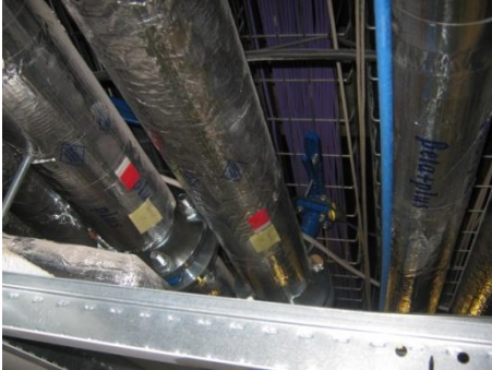
Hot water valves above ceiling tiles
